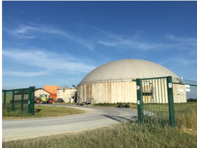
Picture 2: CSTR Semi dry fermentation process based plant operating in Germany
